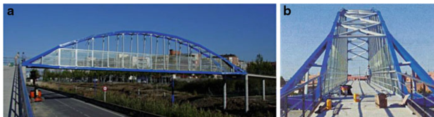
Fig. 11.26 The Lleida bridge: (a) general view (courtesy of Juan Sobrino/PEDELTA) and (b) lateral view [59]
