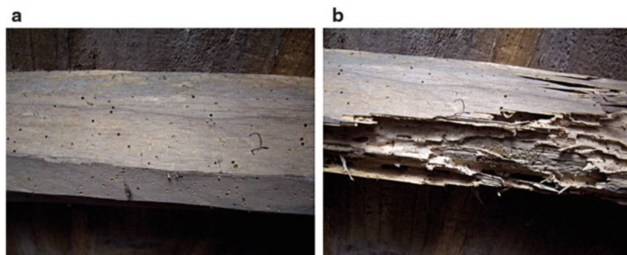
Fig. 12.13 Detail of an eucalyptus beam infected by dry wood termites, before (a) and after (b) the removal of the non-degraded surface wood layer
