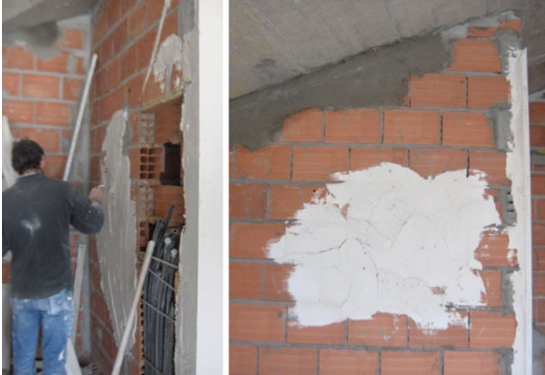
Fig. 3.19 Mechanical treatment of the substrate, eliminating warping and filling cavities with gypsum paste [25]
