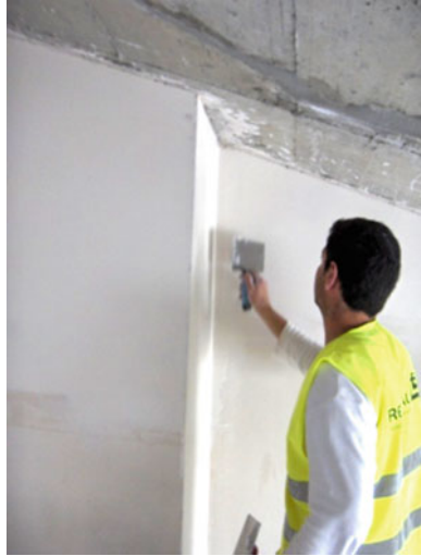
Fig. 3.28 Adjustment of the paste with a corner ruler in re-entrant corners [25]
