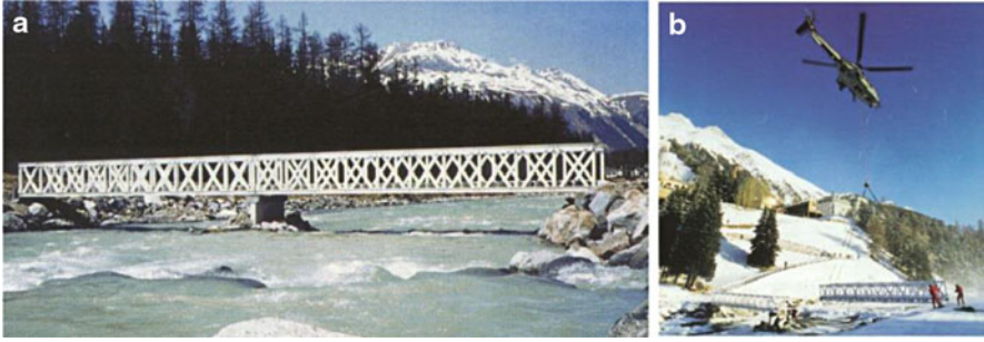
Fig. 11.24 The Pontresina bridge: (a) general view and (b) installation of a span [46]
