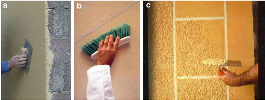
Fig. 2.27 (a) Execution of scraped finish: floating and (b) scrubbing; (c) application of finish in stone in pre-dosed renders [64]
