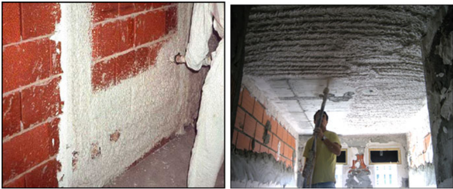
Fig. 3.48 Examples of coating application using spraying devices [27]
