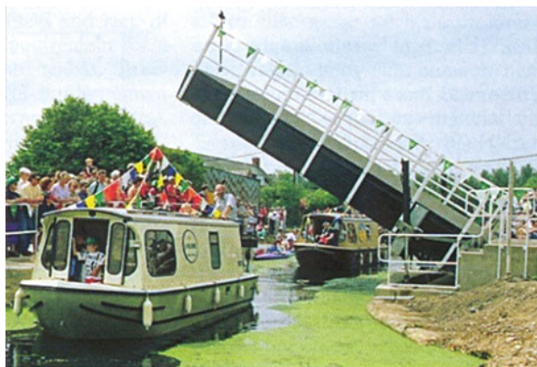
Fig. 11.23 The Bonds Mill Lift Bridge [13]
