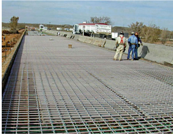
Fig. 11.9 Concrete bridge deck reinforced with GFRP bars
