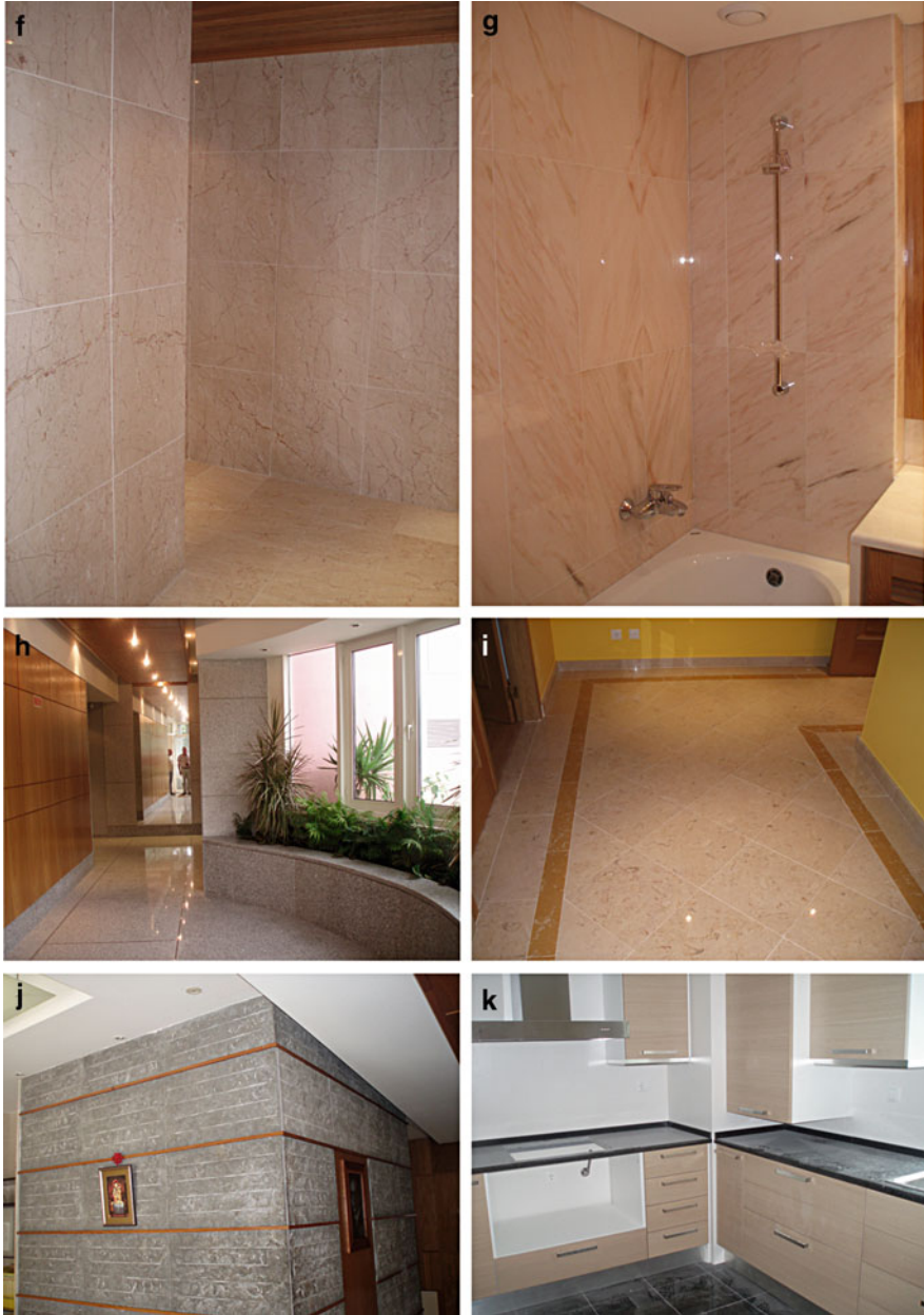
Fig. 9.17 Examples of stone products applications: (a) stairs, (b) exterior cladding, (c) modular tiles for exterior walls, (d) modular tiles for interior walls, (e) slabs for interior cladding, (f) slabs for interior cladding and floors, (g) slabs for interior cladding, (h) slabs for floors and interior walls, (i) modular tiles for interior floor, (j) wood and stone combination for slabs for interior walls, (k) kitchen countertop and modular tiles
