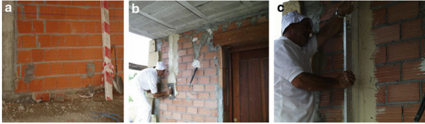
Fig. 2.24 (a) Points and lines technique for rendering mortars: masonry points in masonry before the application of interior plaster; (b) execution of a mortar line; and (c) checking its verticality with a bubble level [64]
