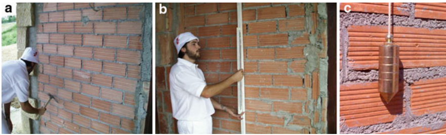
Fig. 2.21 (a) Removal of protrusions; (b) checking planeness with a ruler; and (c) verticality with a plumb line [64]
