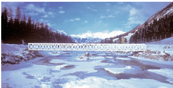
Fig. 11.14 All-FRP Pontresina footbridge [46]
