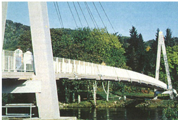
Fig. 11.22 The Aberfeldy bridge [13]
