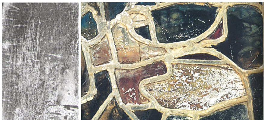
Fig. 8.22 Secondary corrosion: risks and stings in a mediaeval glass from Mosteiro da Batalha (Courtesy of Dr. Pedro Redol, Director of Mosteiro da Batalha, Portugal)
