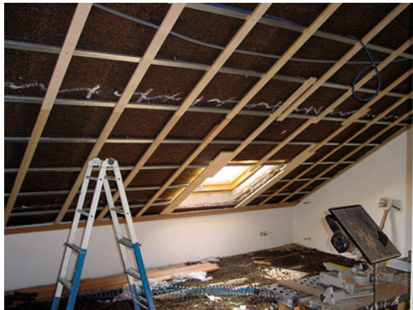
Fig. 13.17 Example of the use of expanded agglomerated cork in roofing
