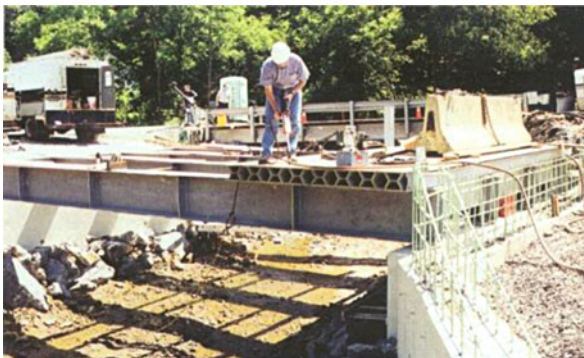
Fig. 11.29 Installation of Superdeck bridge deck (courtesy of Creative Pultrusions)
