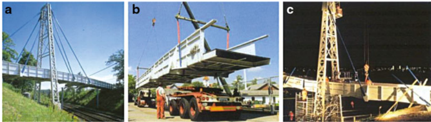
Fig. 11.25 The Kolding bridge: (a) general view, (b) transport of a 27 m long bridge segment and (c) bridge installation during the night [12]
