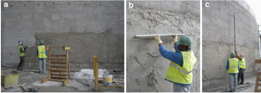
Fig. 2.25 (a) Application of the base coat with spraying device, reference points; (b) pressing and smoothing/levelling the mortar's coat; (c) checking the render's verticality with a reference support [67]
