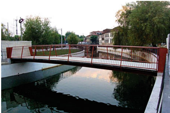
Fig. 11.13 Steel/GFRP hybrid footbridge in Viseu, Portugal
